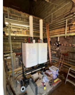
Replacing legacy boilers with energy efficient ones.
